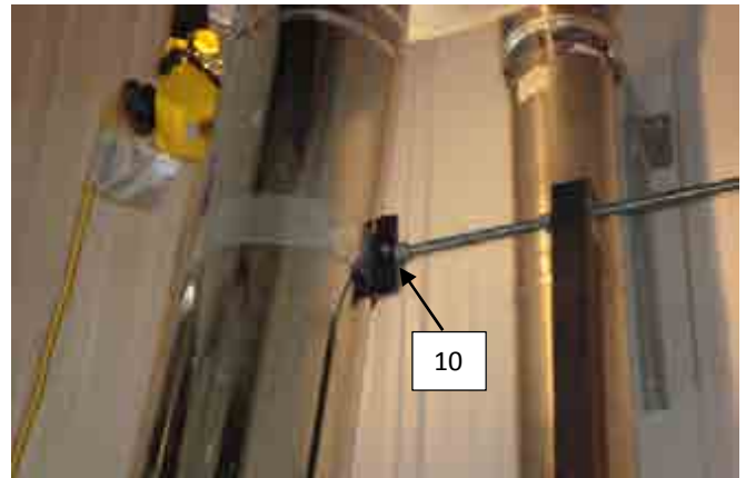
Picture 3.2: chimney support
